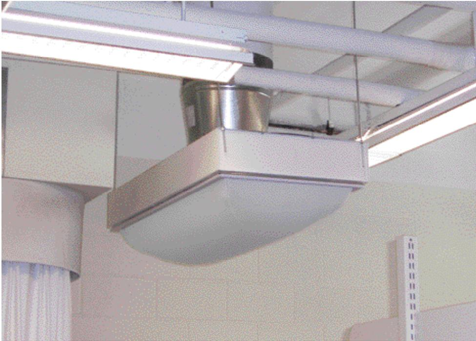
» **Figure 9** A science building at the University of Toronto replaced its original metal diffusers with fabric diffusers for even air flow and slower velocities, while still maintaining the needed cfm's to condition the lab spaces.
