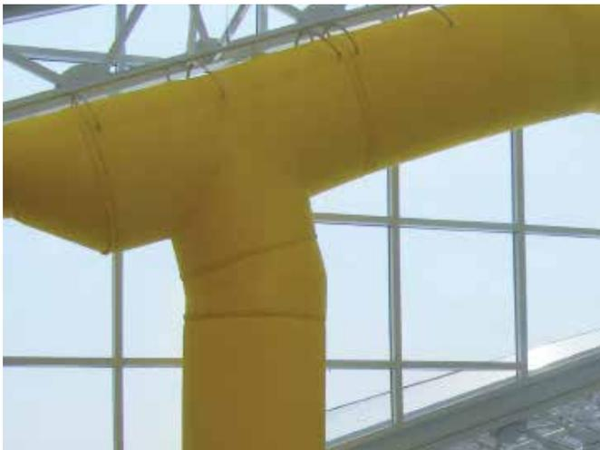
⤵ **Figure 2** Just about any metal fitting shape can be made from fabric. A tee-shaped fitting for textile duct systems made out of fabric is shown here.
