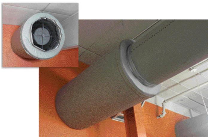
⚡ **Figure 3** The fabric sound attenuators abate noise generated from 14 AHUs ranging from 2,625–4,400 cfm.
