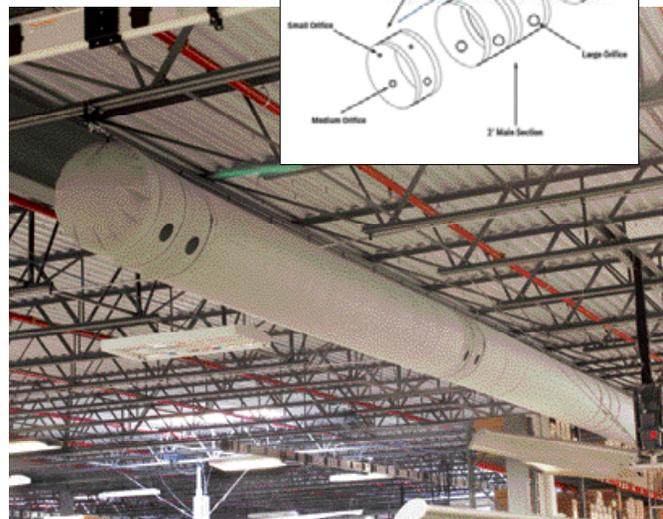
⚡ **Figure 4** Field-adjustable, modular and configurable fabric duct systems are ideal for smaller non-plan/spec projects of approximately 3,000-sq-ft or less.
