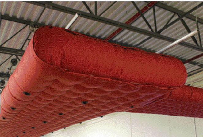
⤴ **Figure 6** The oval-shaped duct for low-clearance applications saves 13–27 in. of head room vs. round fabric or metal duct by spreading out air flow in a structure that ranges from 47–93 in. wide.
