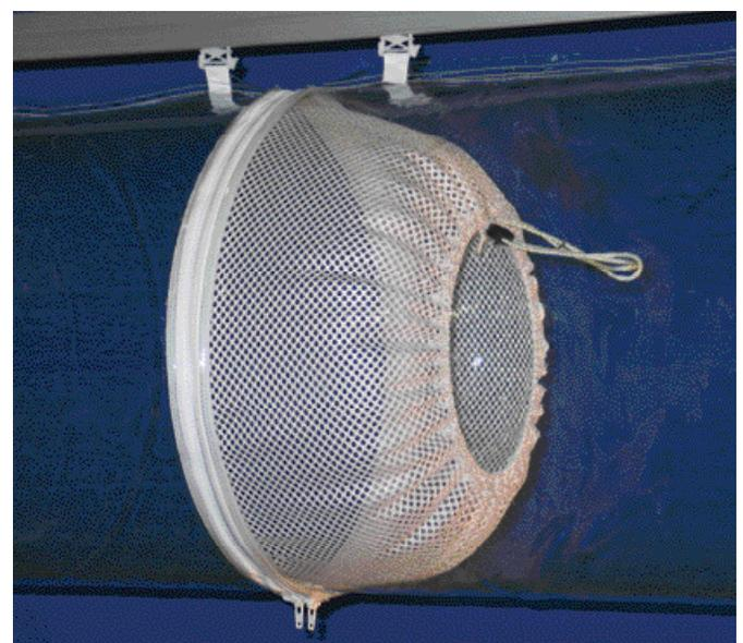
⤴ **Figure 7** The AFD is designed for balancing air flow anywhere throughout a duct run, but is generally factory-set for the inlet to quell turbulence caused by the air handler or its connecting ductwork/elbows.
