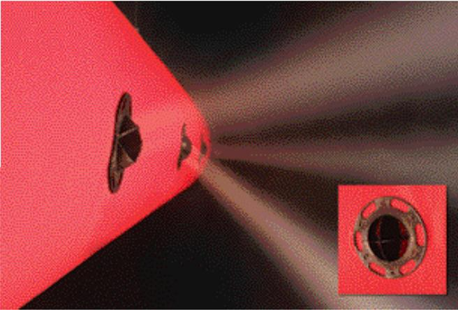
⤴ **Figure 5** Nozzles can be hand-rotated onsite into 10 different notched air-flow angle settings. The hemispheres have a throw range from 50–150 fpm and up to 10–70 ft, respectively.
