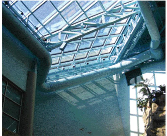
⤵ **Figure 1** Fabric duct has the same types of fittings as metal duct and can be designed to circumvent obstructions or navigate unusual angles.
