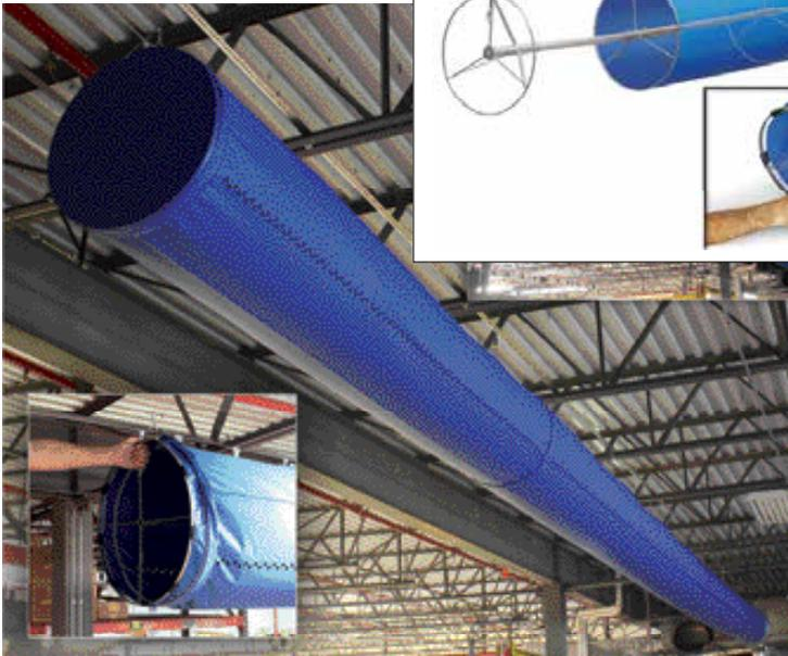
△ **Figure 8** An in-duct tensoning system combines tensioning baskets and internal hoops to offer a perpetual inflated duct appearance.
