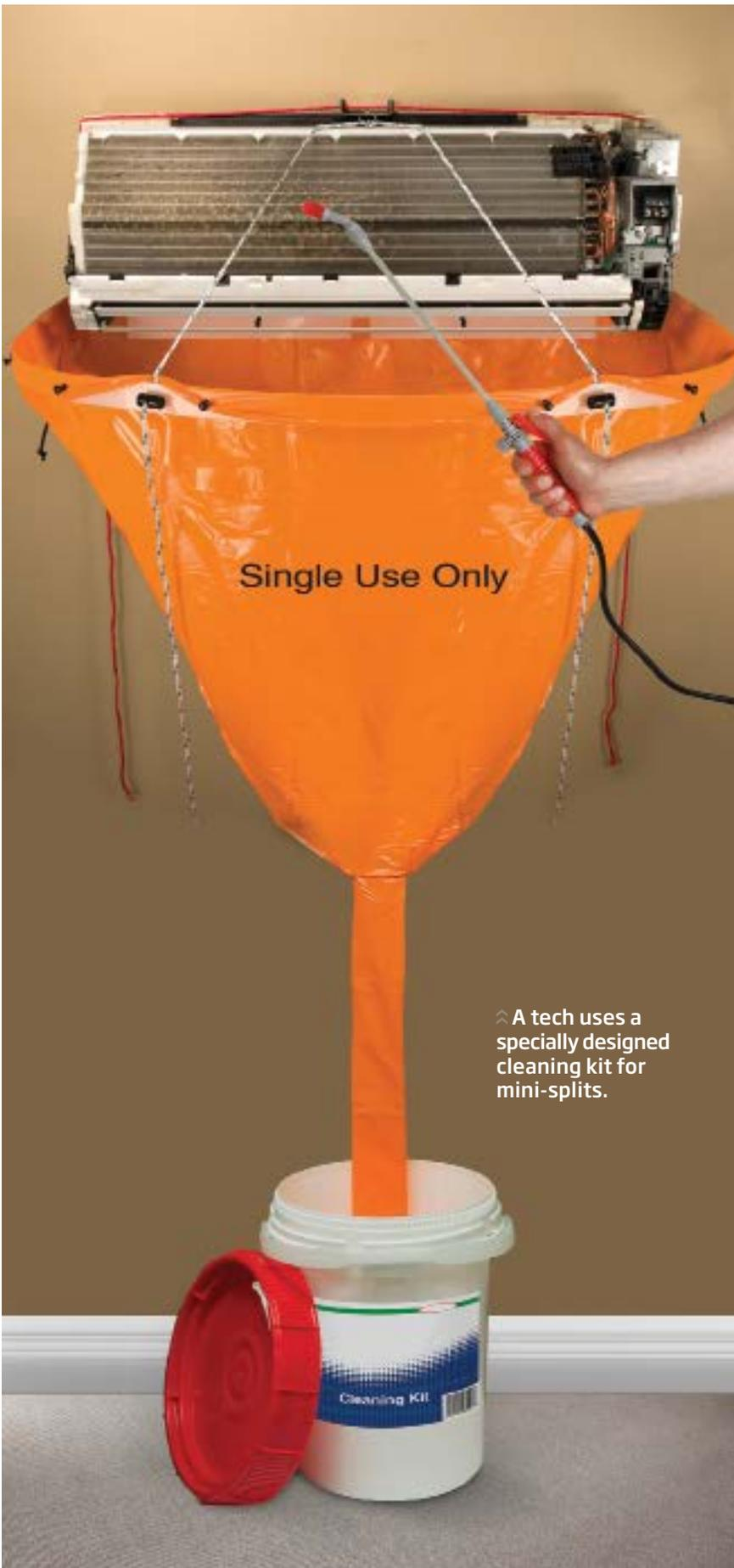
⤵ A tech uses a specially designed cleaning kit for mini-splits.
