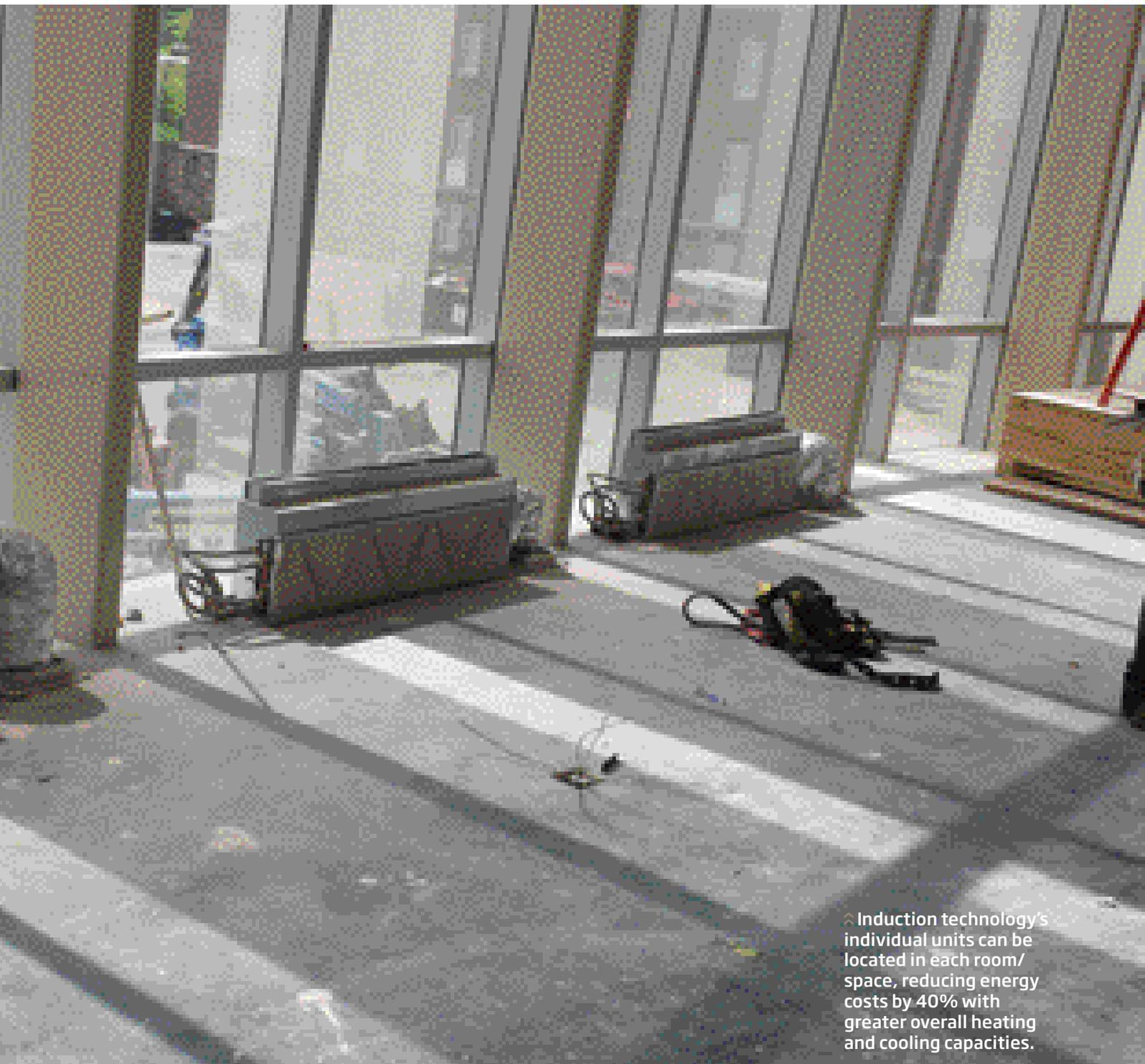
^ Induction technology's individual units can be located in each room/ space, reducing energy costs by 40% with greater overall heating and cooling capacities.
