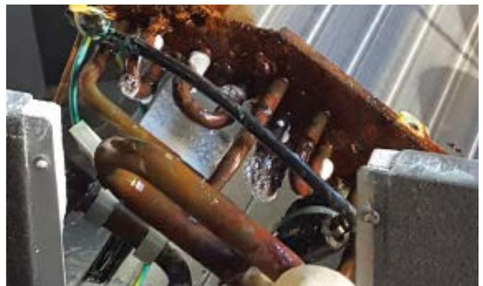
⤴ **Figure 2 Zeroing in on leaks with leak locator bubbles. Technically formicary corrosion cannot be seen with the naked eye so technicians should use bubbles to look for leaks.**
