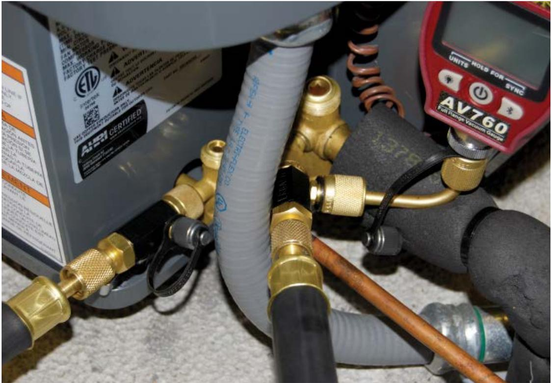
One great way to accomplish this is to use a core removal tool with your micron gauge attached directly to the side port and the evacuation hose connected to the straight port.
