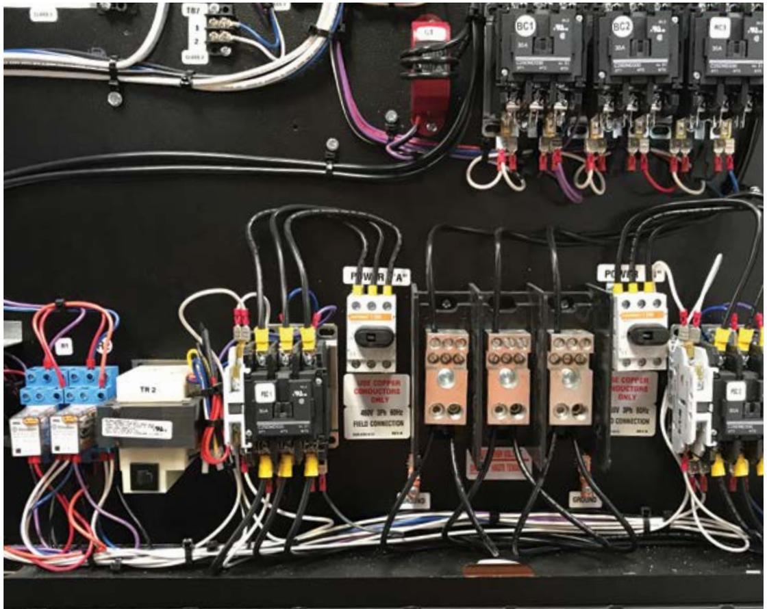
of a phase loss, voltage imbalance and over/under voltage to the unit. The general logic for the phase-loss-monitor is upon a failure being detected, the control voltage is interrupted. This will prevent operation of the unit until the fault is corrected. Most of these devices can be added after the units have been installed and operating.
