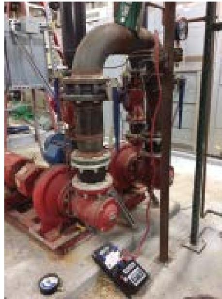
« A hydronic differential pressure meter is used to measure the actual pump or system head.
