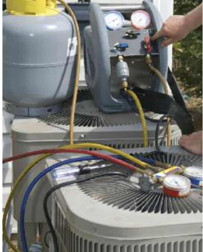
**Because R-410A operates at a much higher pressure than R-22, technicians should have specific recovery equipment, hoses, gauges and other related equipment dedicated for use with hydrofluorocarbons.**
