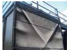
ging up the system. The washable, ultraviolet-protected filter reduces equipment maintenance, downtime, and frequent and labor-intensive chemical cleanings, and it requires no system modifications or electrical hookups. Custom made to the air-intake perimeter, a variety of design features allow for easy and secure filter attachment. **Circle 18 on the reader service card.**
