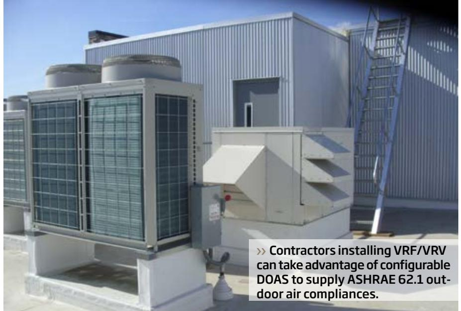
» Contractors installing VRF/VRV can take advantage of configurable DOAS to supply ASHRAE 62.1 outdoor air compliances.
