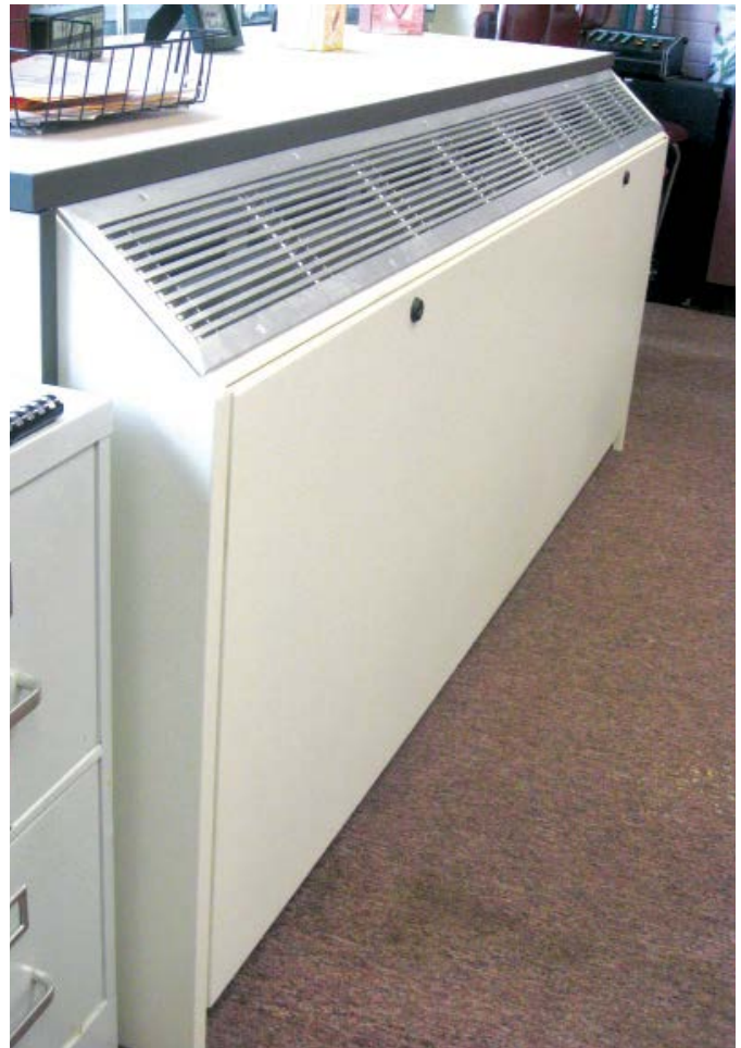
⚡ A VRF/ERV drop-in replacement used in a school retrofit.
