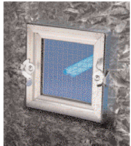
Figure 3 Access view port doors allow techs to easily replace lamps.
