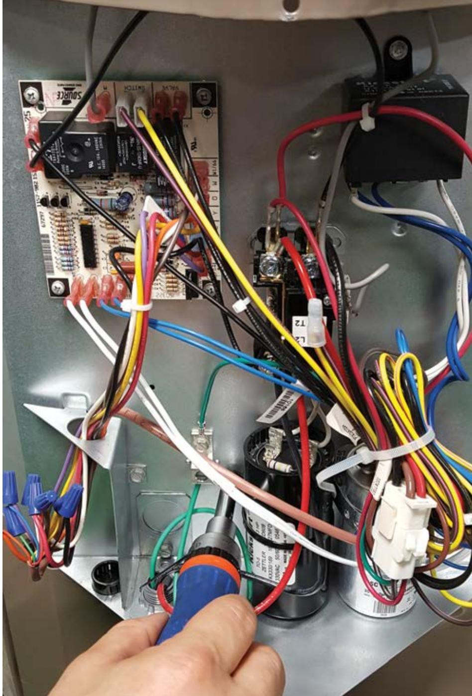
« Securing the start capacitor in the electrical control compartment is simple with the strap included with the two wire kit.
