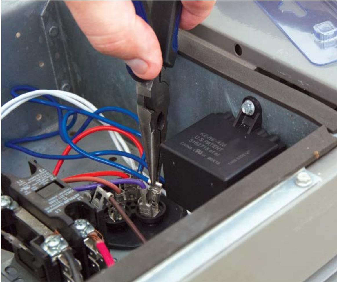
« Wiring a two wire kit into the system is easy. Simply connect one blue wire to both sides of a single run capacitor or to the “common” and “herm” terminals of a dual run capacitor. Reversing the blue wires does not change the functionality of the hard start kit.
