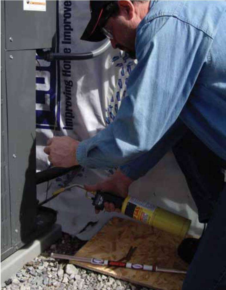
« From residential units to those found in industrial/commercial applications, properly brazed connections eliminate moisture from systems and help ensure efficient, effective equipment operation.
