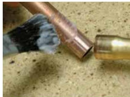
« **Image 1.** Since flux contains moisture—the enemy of an HVACR system—techs should keep excess flux from inside the lines using a brush to apply a thin coating of the substance to copper tubing.
