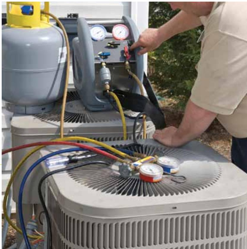
» Because R-410A has a much higher pressure than R-22—about 50% or more higher under the same temperature conditions—technicians must have pressure gauges, hoses and recovery equipment rated to deal with those higher pressures.
