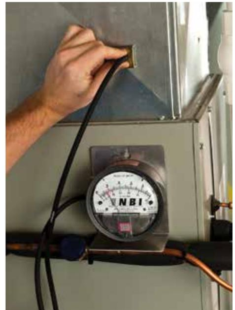
⚠ If you see duct pressures that exceed 0.10 in. wc, rest assured there is a restriction somewhere on that side of the duct system.
