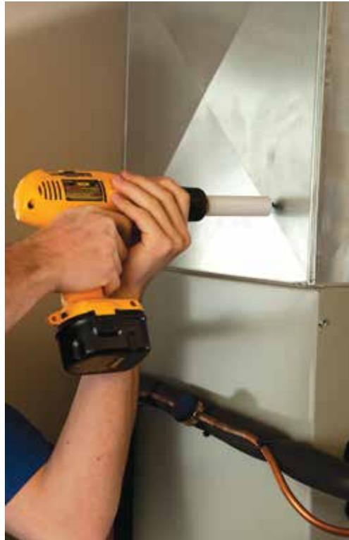
« When drilling test holes in equipment, using a drill bit sheath or step bit will help to avoid damage to electrical components, drain pans, coils and heat exchangers.
